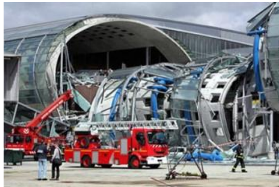
Figure 2-4. Collapse of Terminal 2E of the Charles de Gaulle Airport, Paris, France (2004) 7
