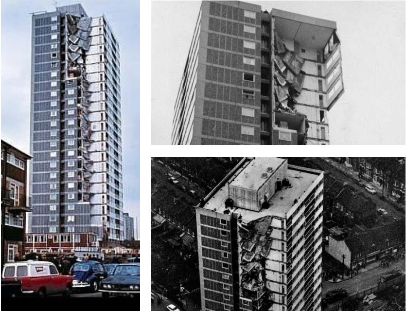
Figure 2-1. Collapse of Ronan Point Building, London, UK (1968) 4
