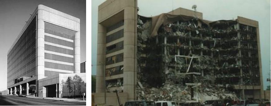
Figure 2-2. Collapse of the Alfred Murrah Federal Building, Oklahoma City, USA (1995) 5
