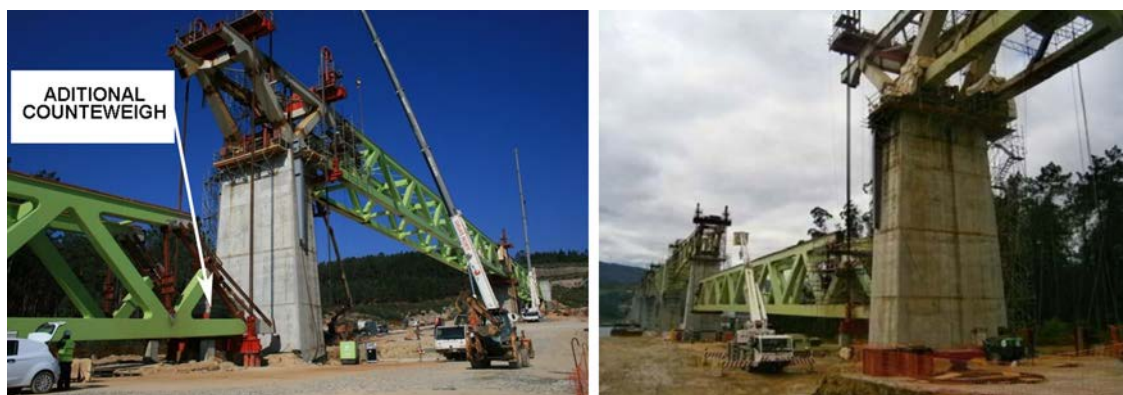
Figure 28. Hoisting sequence for spans 11 (left) and 10 (right).
