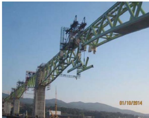
Figure 43. Hoisting the joining segment for span 8.
