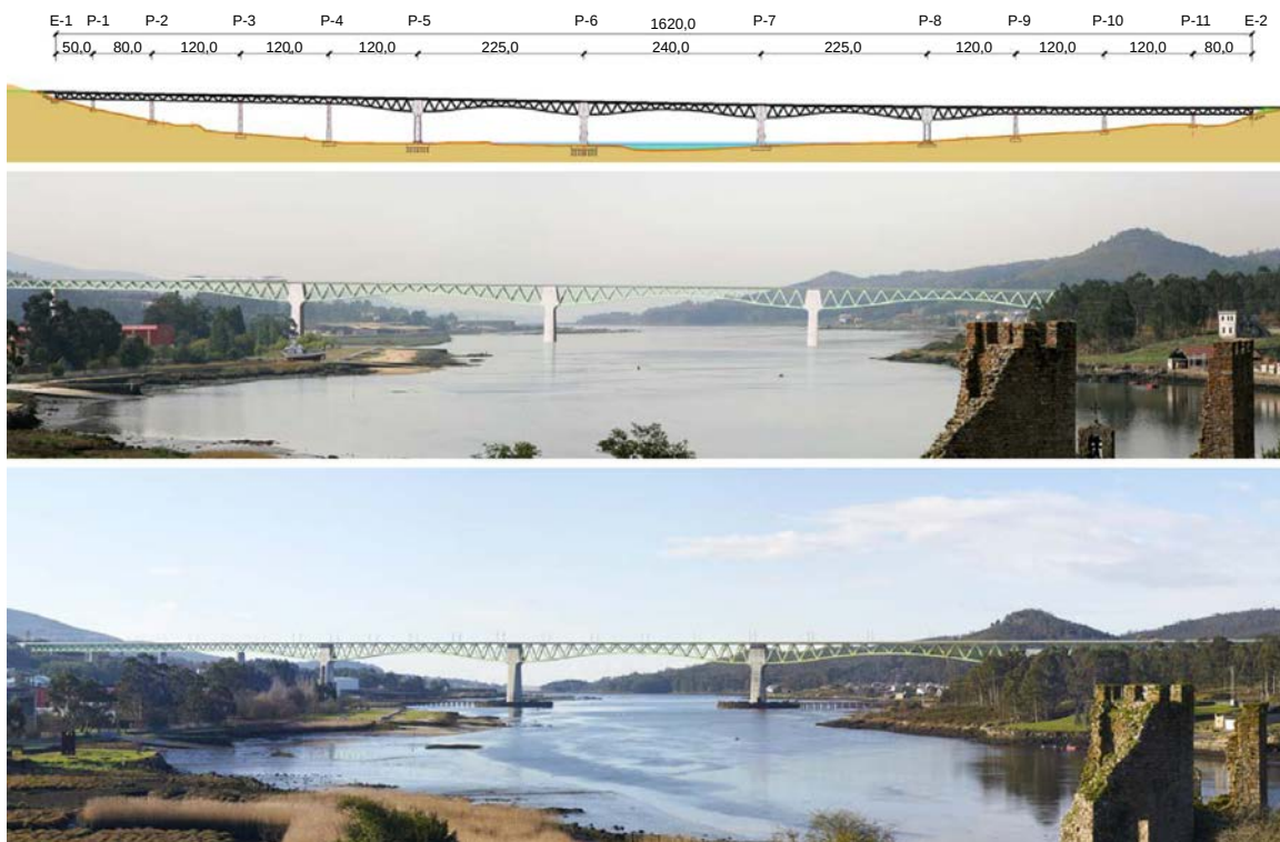
Figure 1. Elevation drawing, simulation and photograph of the finished viaduct over the River Ulla.
