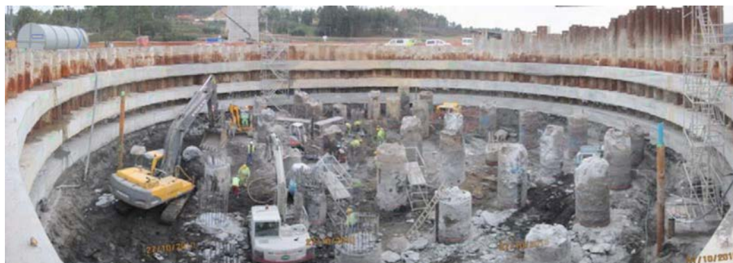
Figure 9. Cutting down P5 foundation pile heads.
