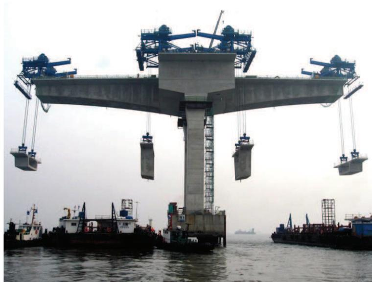
**Figure 3:** Construction of a maritime bridge using precast concrete box girders
