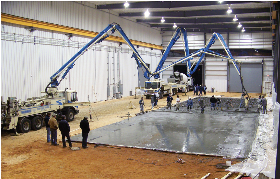
Fig. 4.4.2—Truck-mounted boom pump.
