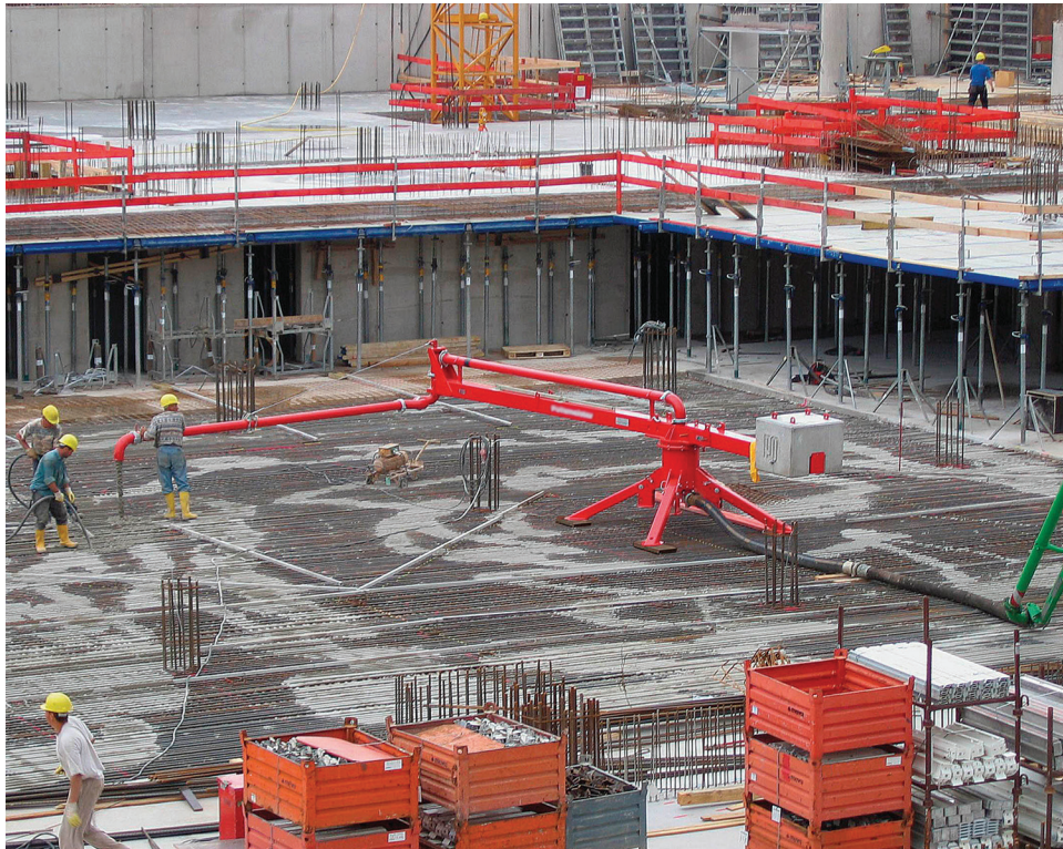
Fig. 6.2b—Rotary distributor placing booms.
