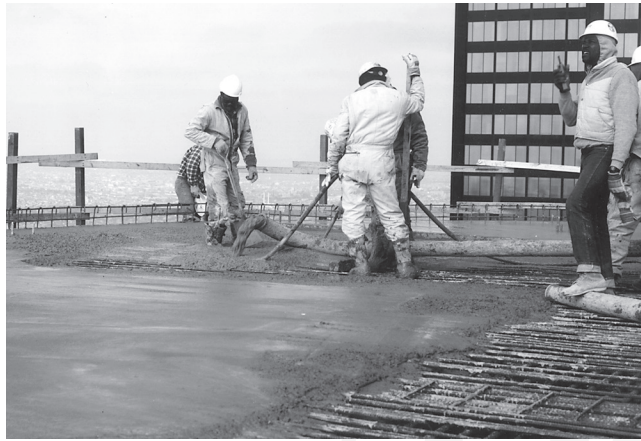
Fig. 6.2a—Material placement with flexible hose at end of rigid pipeline.
