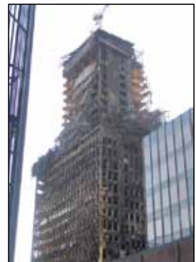
Figura 10.9. Torre Windsor. Madrid.
