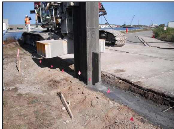
Photo 4 - Excavated trench used to contain excess slurry.
