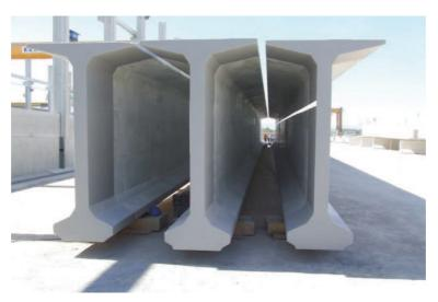
Figure 2: I section beam. One of the most common profiles to design and build the deck bridge
