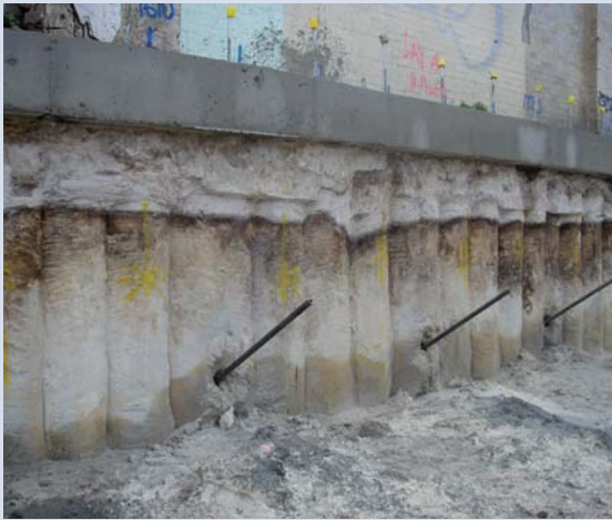
Excavated SMW retaining wall, Sydney, Australia
