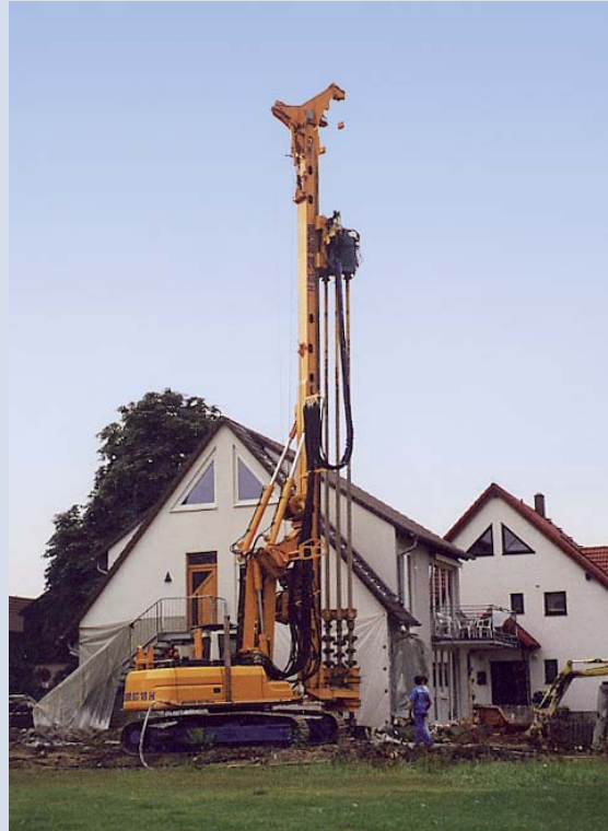
Cut-off wall with BG, Oberhausen, Germany
