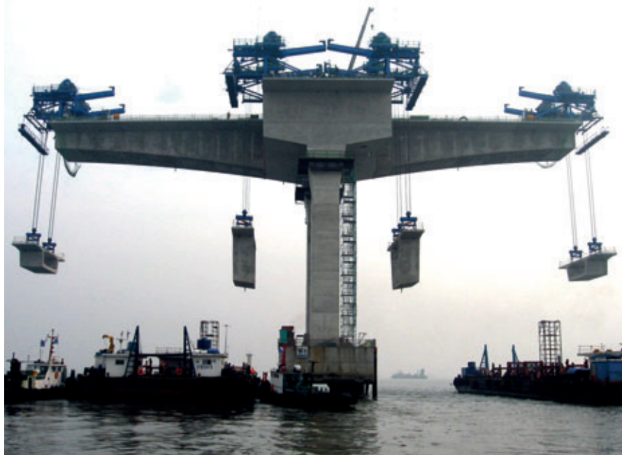
Figure 4: Construction of a maritime bridge using precast concrete box girders
