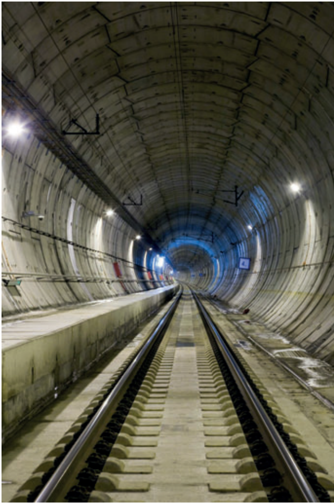
Figure 2: Sleepers and segmental linings play a essential role in the construction of railway lines and tunnels as it is currently happening in two of the biggest works at the new crossing of the Bosphorus Strait in Istanbul and the new Crossrail line in London
